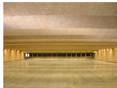
SPECIAL OPERATIONS CMD Ft. Bragg, Ft Carson, Ft Campbell, Ft Lewis; sole sourced to meet USACE ASTM RT60 1.3 seconds reverb time.
