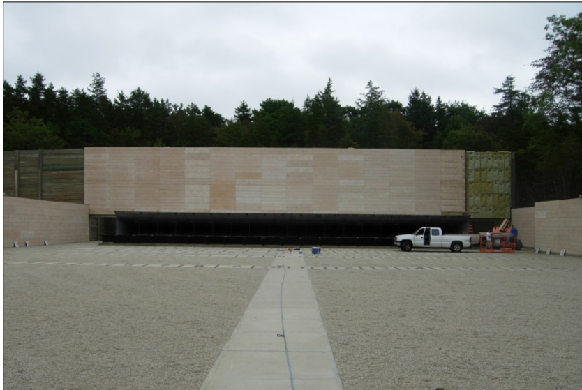
Monmouth County range had a 10dB or 50% noise reduction with the Troy System
