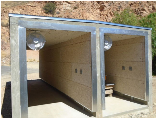
Customized acoustic shooting stalls can reduce noise levels by as much as 10 dB
