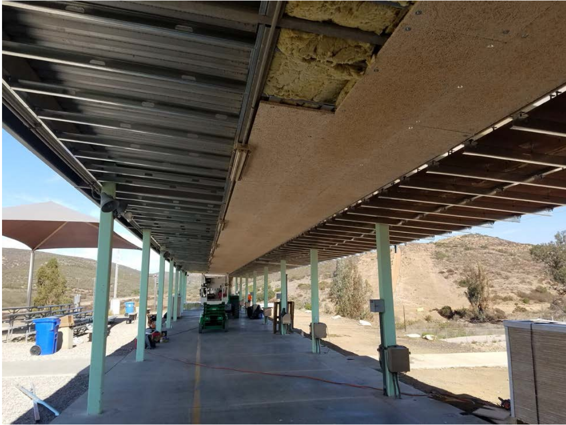
Metal canopy with the Troy System lowered the average sound pressure levels
